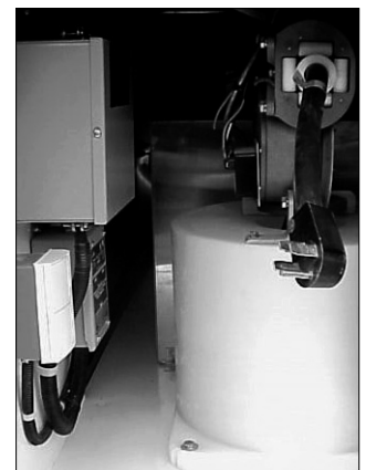
Power Cable Reel
